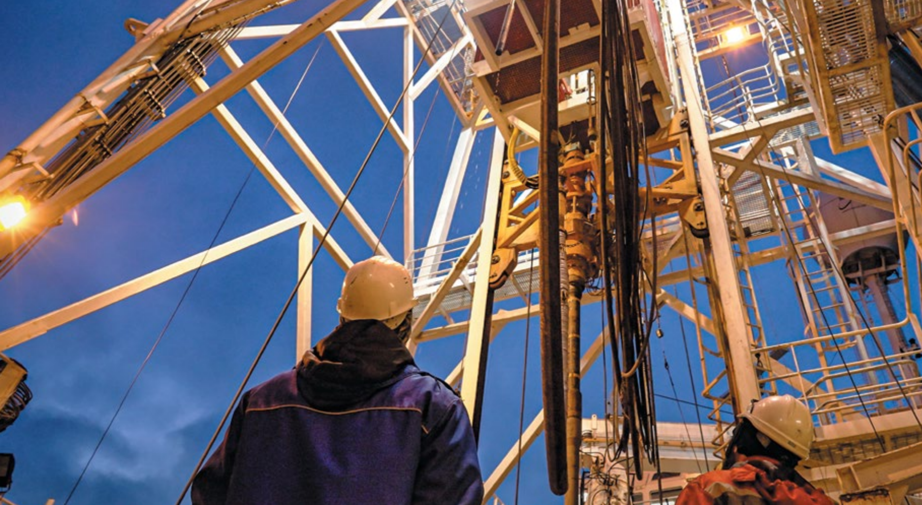
Drilling rig on the vessel Bavenit
